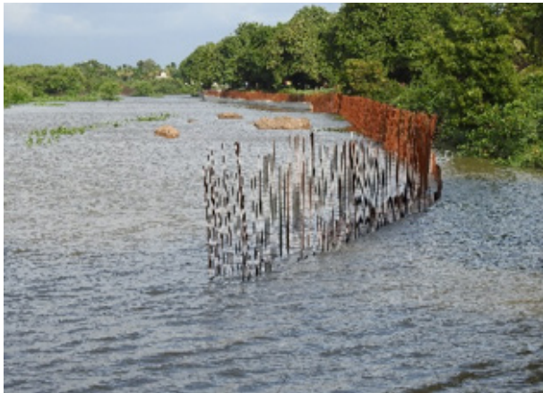
Image 8. The submerged containment wall during the monsoon season. © G. Parameswaran
