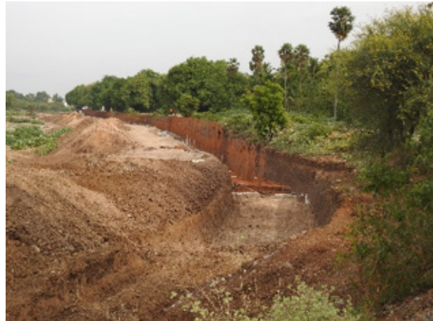
Image 7. Building of the containment wall in the wetland for road expansion during the dry season. © G. Parameswaran.
